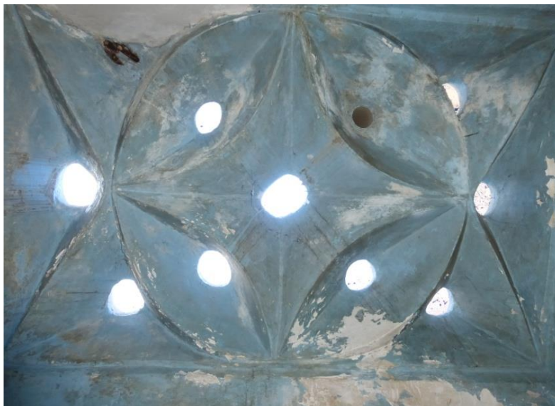
Fig. 9: The ribbed vault of the hammam.
