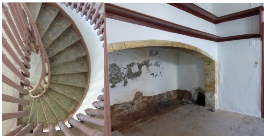
Fig. 6: The main staircase.
